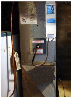
7. Plug the UV cable from the control box into the UV tube. Plug the DC plug from the desktop adapter into the control box. Make sure the power switch is turned off and then plug the desktop adapter into the wall receptacle.
