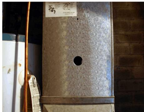
4. Place the UV tube bracket plate over the hole with the black plastic tube mount in the center of the hole with the stickers on the outside as shown. Mark the 4 holes in the corners, Remove the mounting plate and pre drill the 4 holes with a 3/32" or smaller drill bit.
