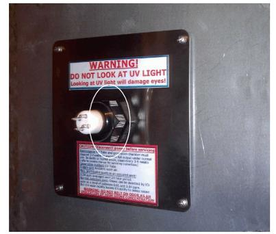
2. Remove the tube by carefully sliding it out.
