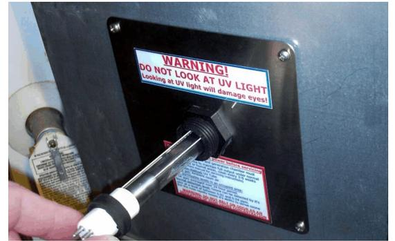
3. In a normal situation the tube will just need to have the dust removed. This can be done using a dusting cloth such as a Swiffer® duster or Swiffer® cloth.
